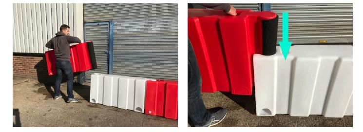
Ensure that each FloodStop unit is fully assembled. The key way should be **fully pressed down**. The gasket should be in contact with the ground terrain.
